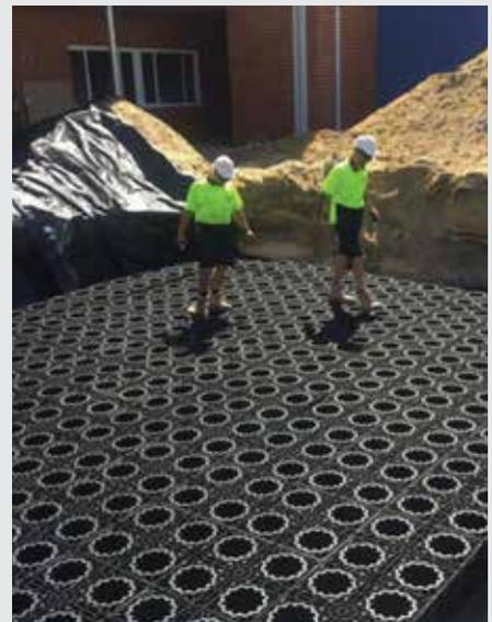
**StormBrixx® SD and StormBrixx® HD with silt trap is ideal for retention and detention applications**
