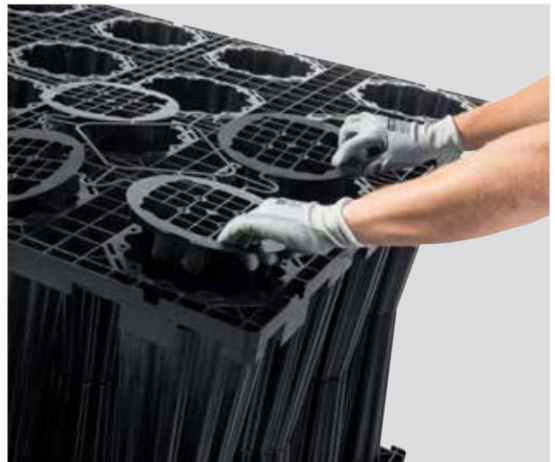
Polypropylene top covers are added to the top layer of the tank to fill the openings of the pillars and to ensure consistent support for the cover fill material.
